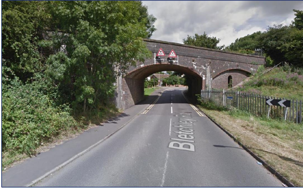
Figure C.4: Limited Clearance bridge on Bletchley Road (HGV access route)
